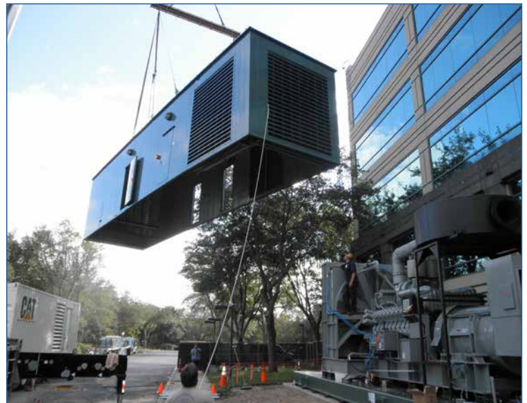
2.5MW Diesel Generator Installation
