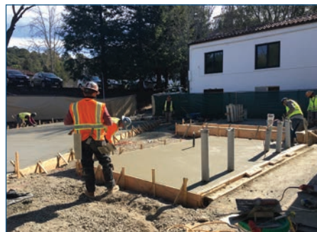
Construction of Concrete Pad
