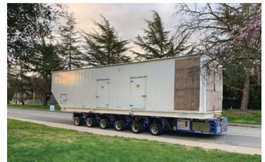
Delivery of Caterpillar 2.5 MW Generator
