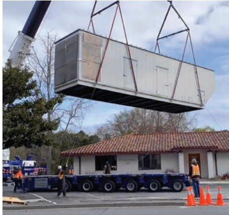
Craning of Caterpillar Generator
