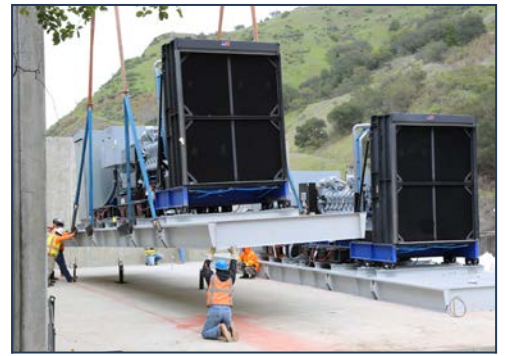
Craning of Generators
