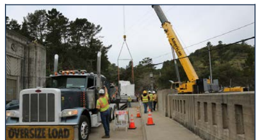
Delivery of Generators to Caldecott
