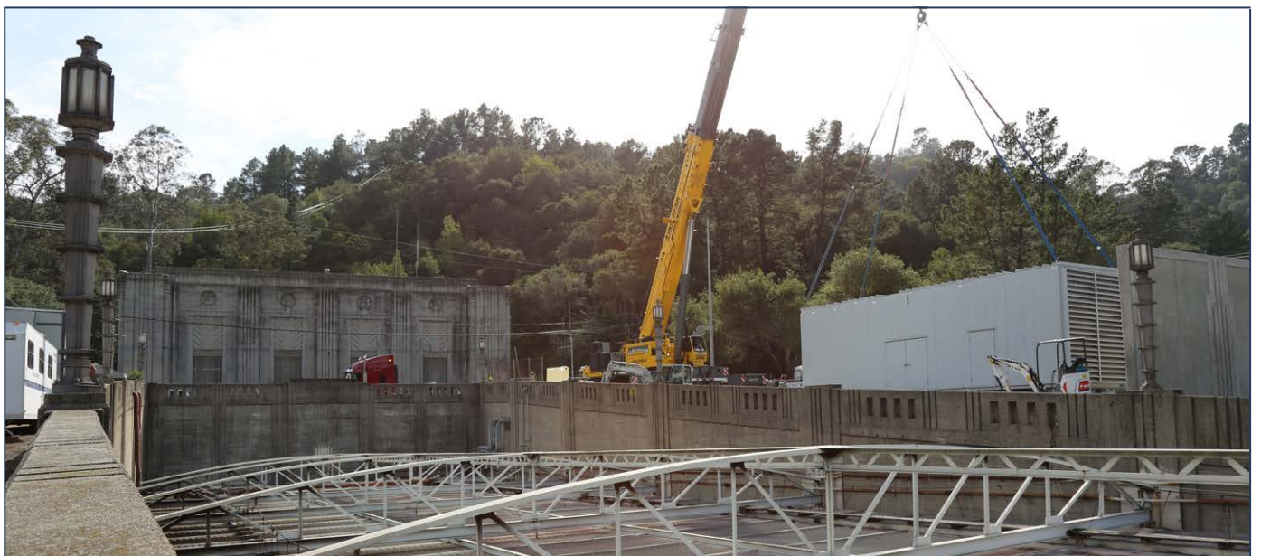
Caldecott Tunnel, Oakland, CA.
