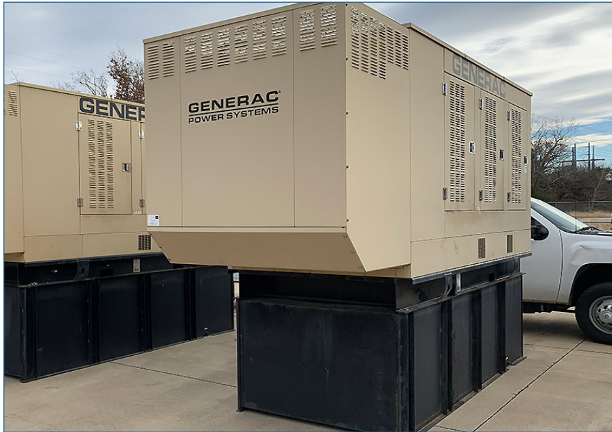
Generac 400 kW MD400 Standby Diesel Generator
