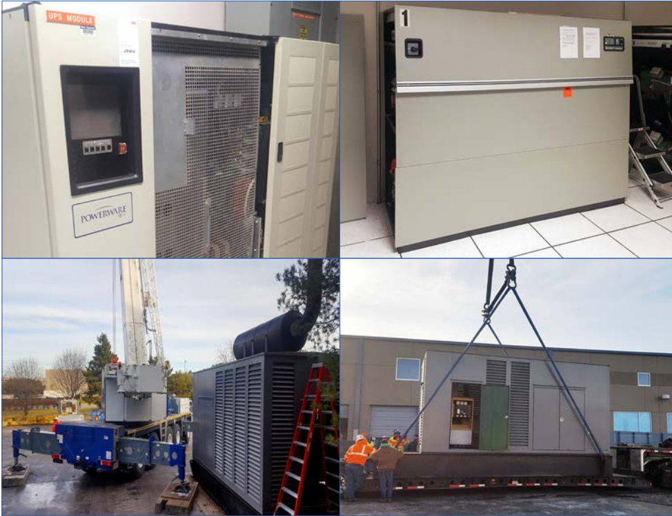
Asset Recovery and Decommission: UPS, Precision Cooling and Generator
