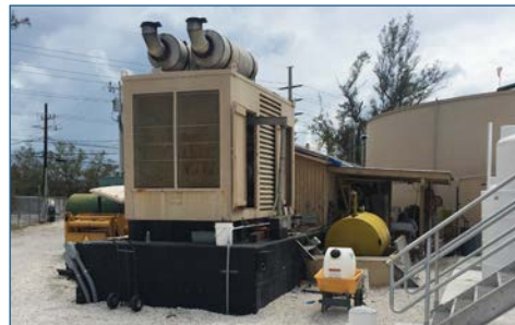
Kohler Genset Removed
