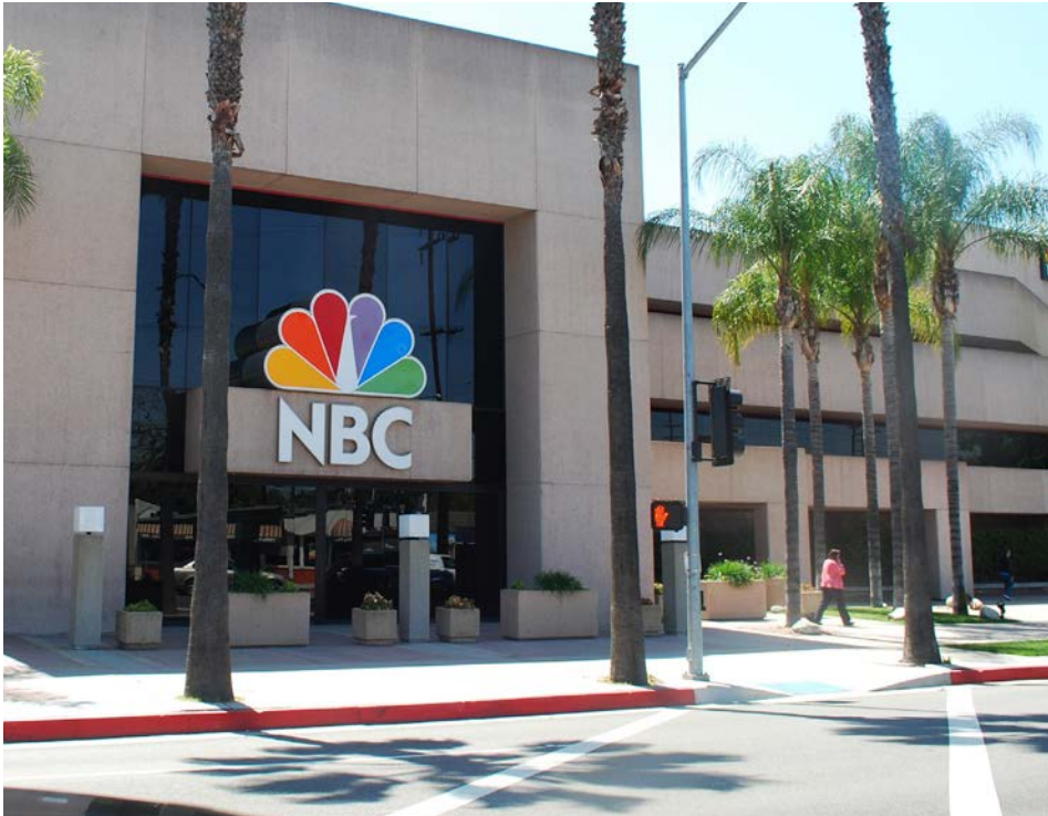
UPS Replacement and Asset Recovery at NBC Studio in Los Angeles
