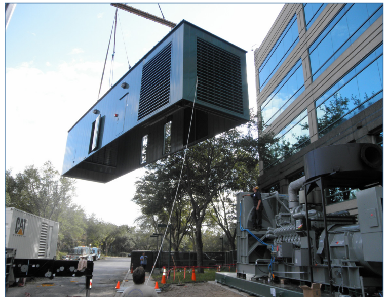
2.5MW Diesel Generator Installation
