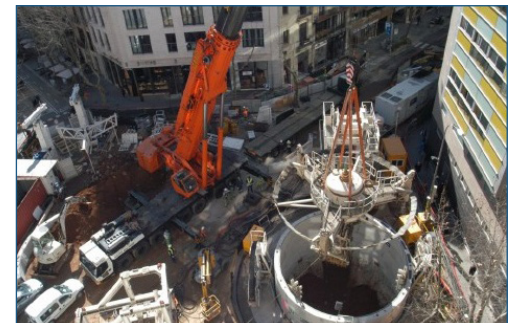
Downtown Macro CAES in Bore Construction
