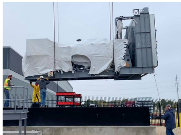
Data Center Generator Installation
