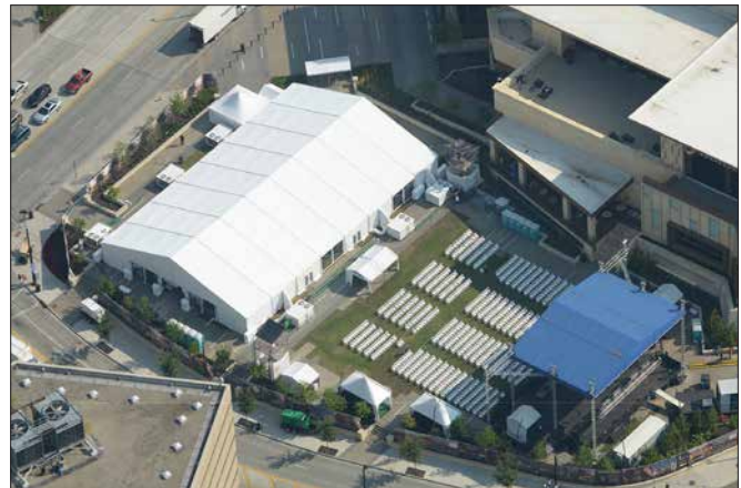
Turnkey Power Generation and Project Management
