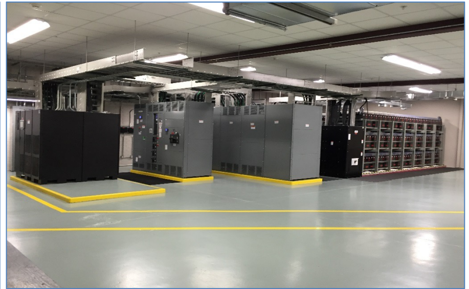
Site completed with new UPS Systems
