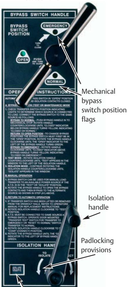
**Fig. 9:** Bypass-Isolation Switch user interface
