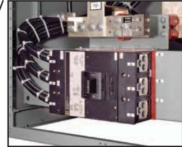
**Fig. 10:** Ground and neutral disconnect links
