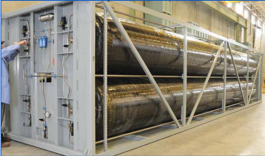
Micro containerized CAES systems for the delivery of stored energy volume for peak hours.
