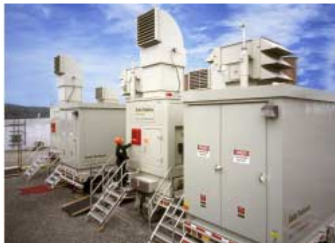
Sited Configuration of Taurus 60 Mobile Power Unit
