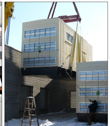
Deinstallation, Rigging & Removal
