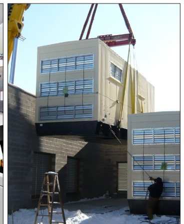
Deinstallation, Rigging & Removal
