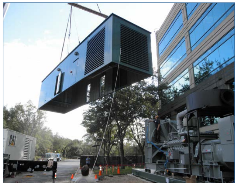
2.5MW Diesel Generator Installation
